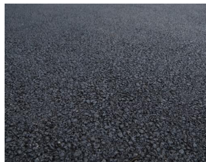
Hot rolled asphalt
